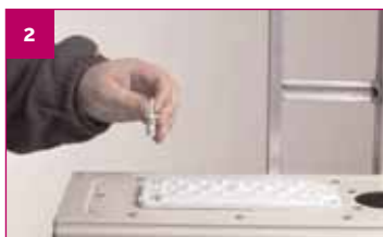
2 Push the plastic rivet or metal screws through the Multigate and the wall of the box.
